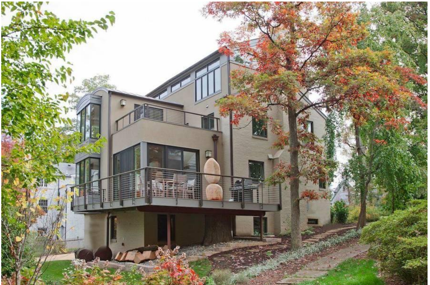
Exterior, Arlington House
